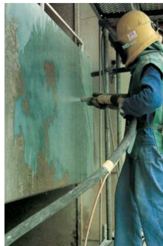
Renovácia betónu Concrete refurbishment
